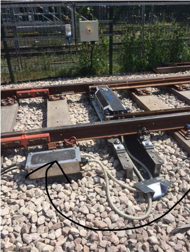
*Frequency converter shown here outside of hollow steel bearer – will be placed within allowing a fully tampable switch*
