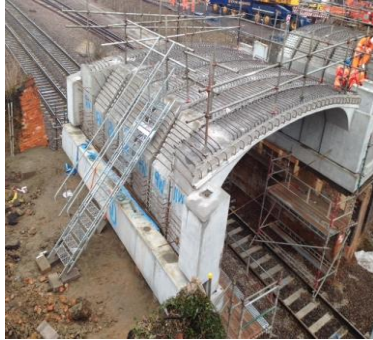
Civil and structural engineering Track design and renewal
