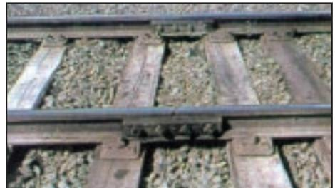
The sleeper spacings are wrong, one tight and open joint indicates frozen fishplates.
