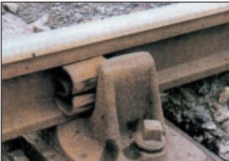
This steel key does not fit correctly. The ballast is very dirty.
