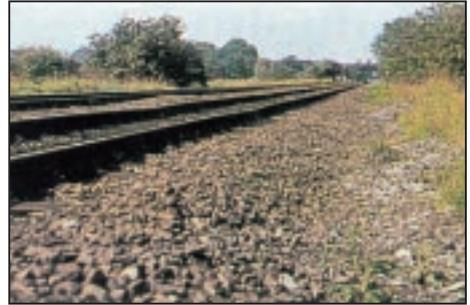
Dipped joints such as this will cause the rails to be driven forward.
