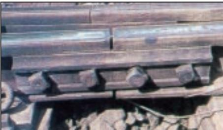
The heel joint at a cast AMS crossing. No TJ plates and a mixture of bolts, permitting the plain rails to move.
