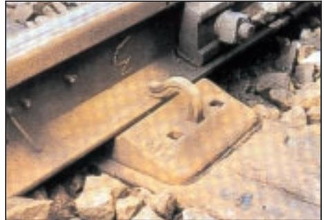
This spike is ineffective; the rail is not tight in the baseplate and the baseplate is shuffling.
