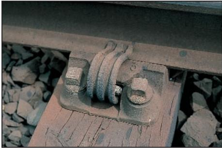
Mills rail clips fit into a pocket cast into the baseplate and whilst the clip may be retained in the pocket, it is possible that some or all of the clip toe load can be lost and the clips rattle during the passage of a train. In these circumstances it will be necessary to either fit toe shoes (wedges) to the clips or to replace the clips.
