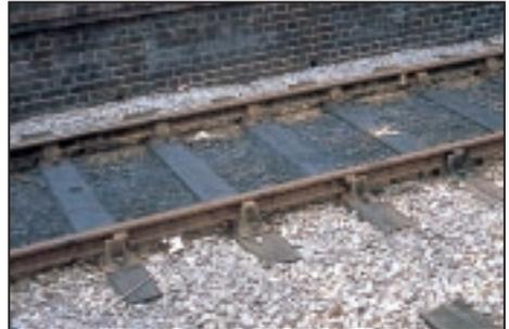
Keys correctly driven in alternative directions
