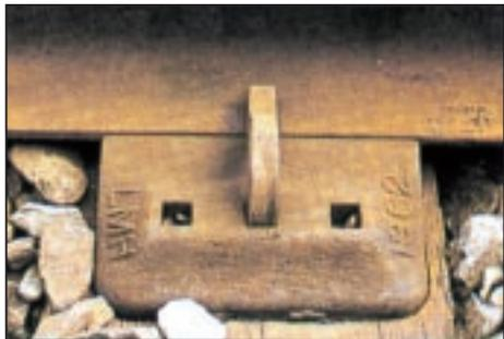
The marks on the top of the rail foot, to the left of the spike and to the right of the baseplate indicate that the rail has been pulled back at least twice.
