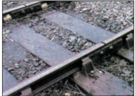
Two bolts in four hole fishplates, wet beds, lack of ferrules will all lead to creep.
