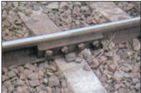
A joint on top of the sleeper. When was it last lubricated or pulled back?
