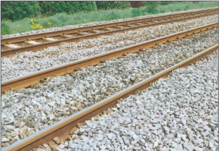
Figure 10 Excess ballast must be removed quickly to allow inspection
