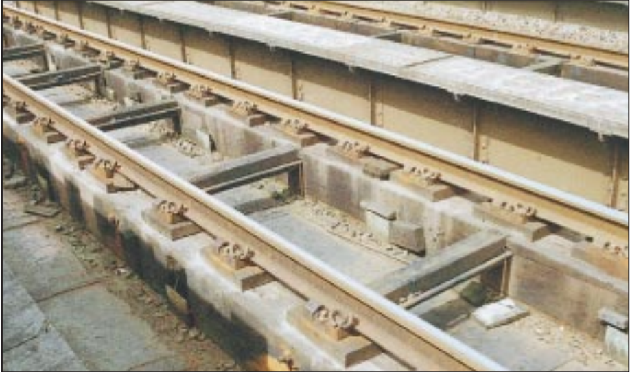
Figure 11 Longitudinal timbers require detailed attention
