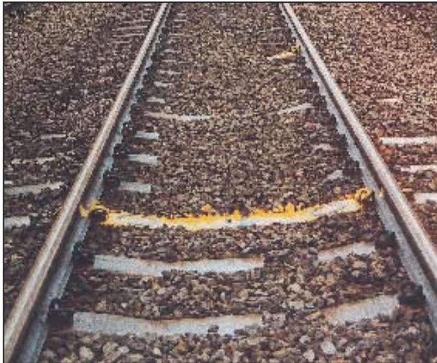
*Photograph- transition curve with cant marking*
