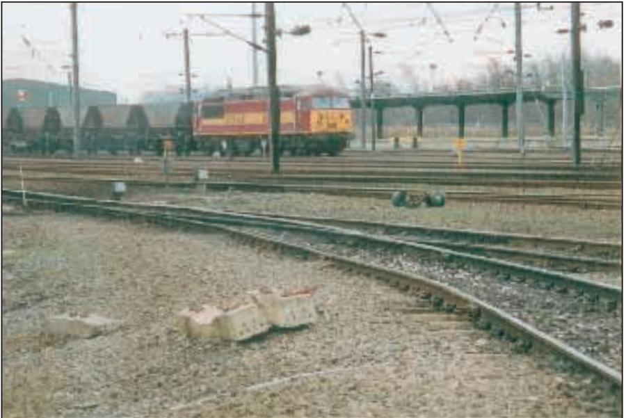
*Photograph - derailment risk twist fault in S&C*
