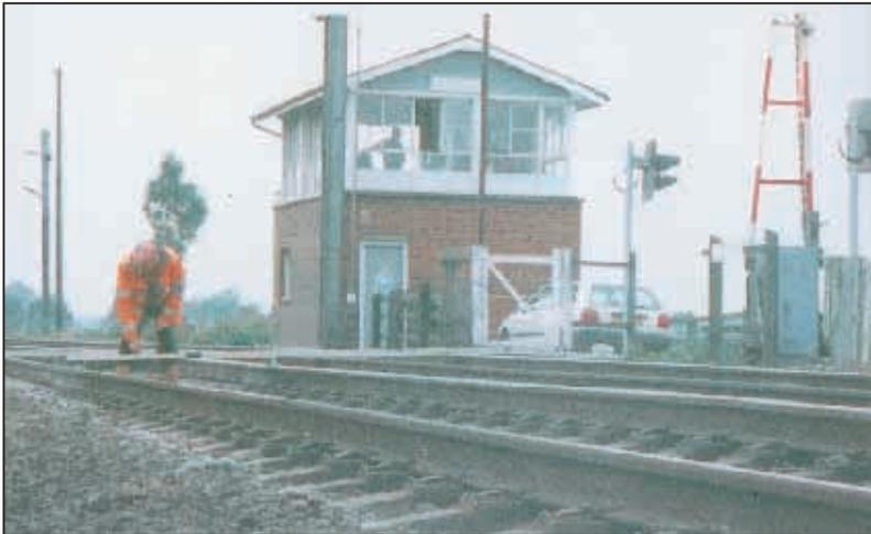
*Photograph - twist fault measured at a Level Crossing*
