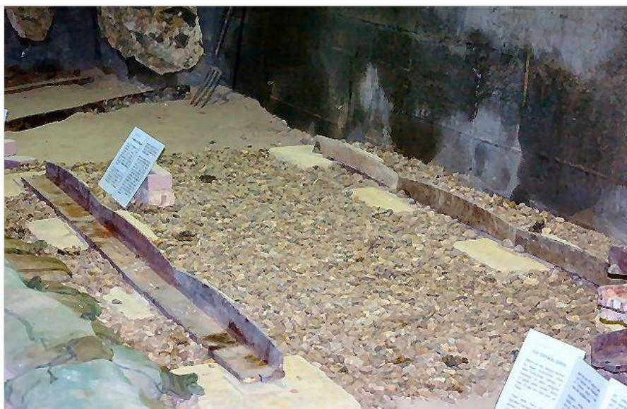
Image 3: L section plate way Croydon Merstham Godstone Railway
