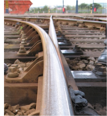
Tramway (embedded and ballast) and NR Switches
