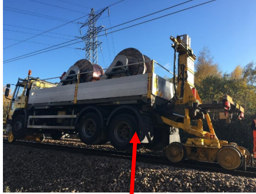
Contact and catenary wire installed in normal manner
